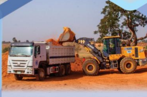
Construction of the 35km World Bank sponsored Access Road projects (RAAMP) in plateau state
